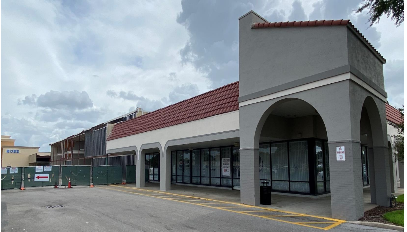
Front facing north (Marshalls currently under construction)
