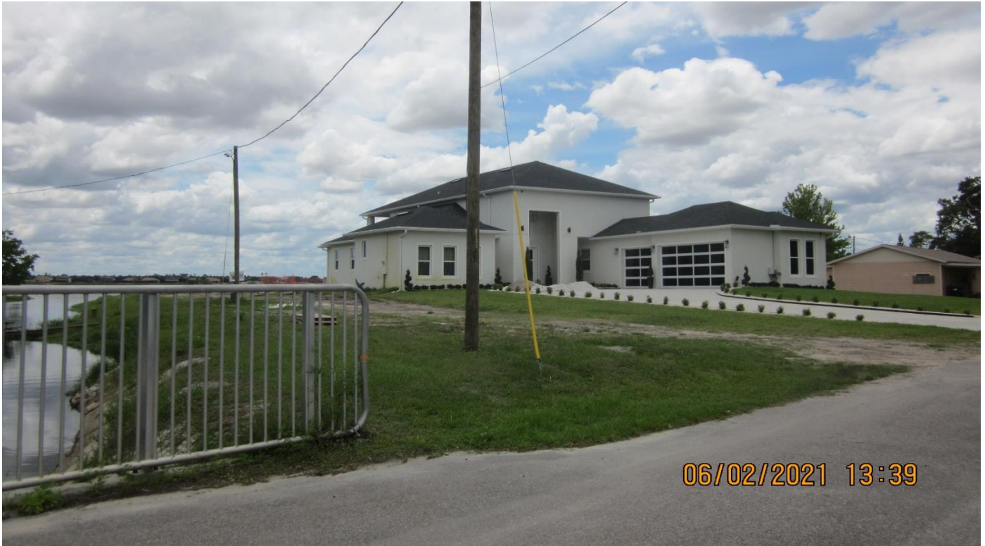
East side of subject property facing south
