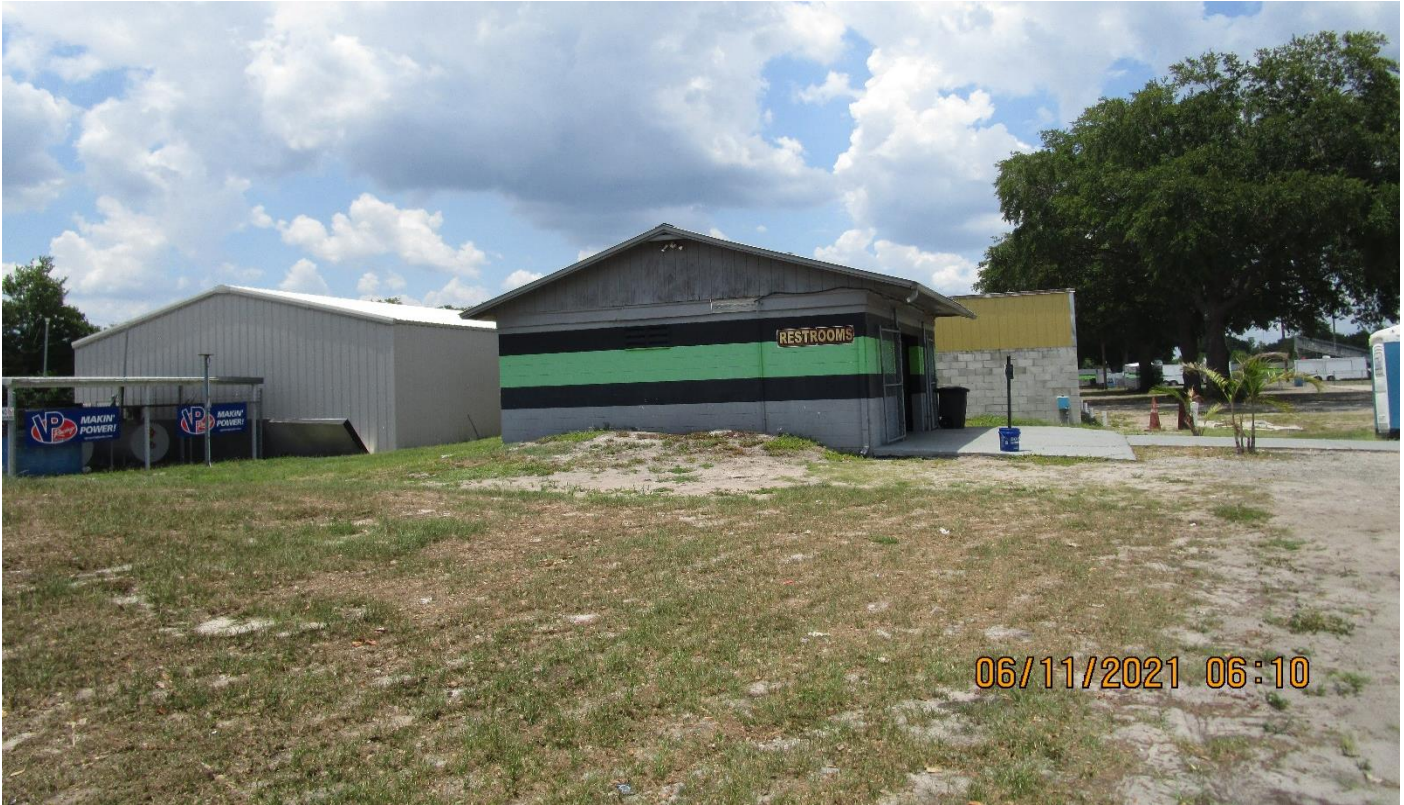
Storage Building 11, Restroom Building 8, unfinished Restroom Building 10 facing northwest
