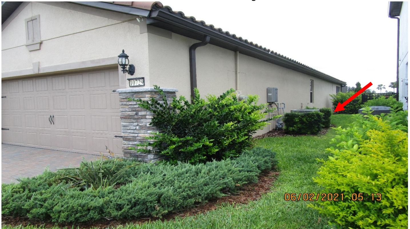
Side-Generator location facing north
