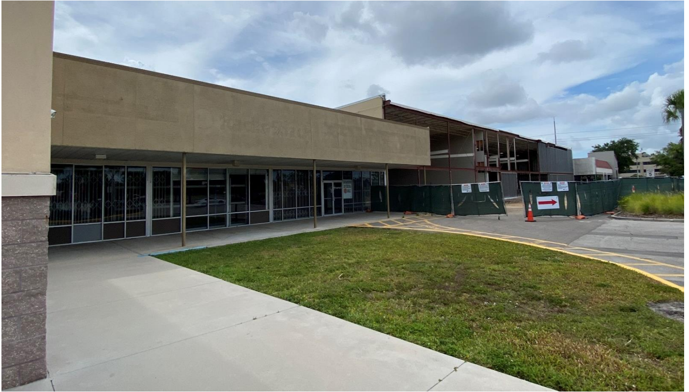
Front facing south (Marshalls currently under construction)
