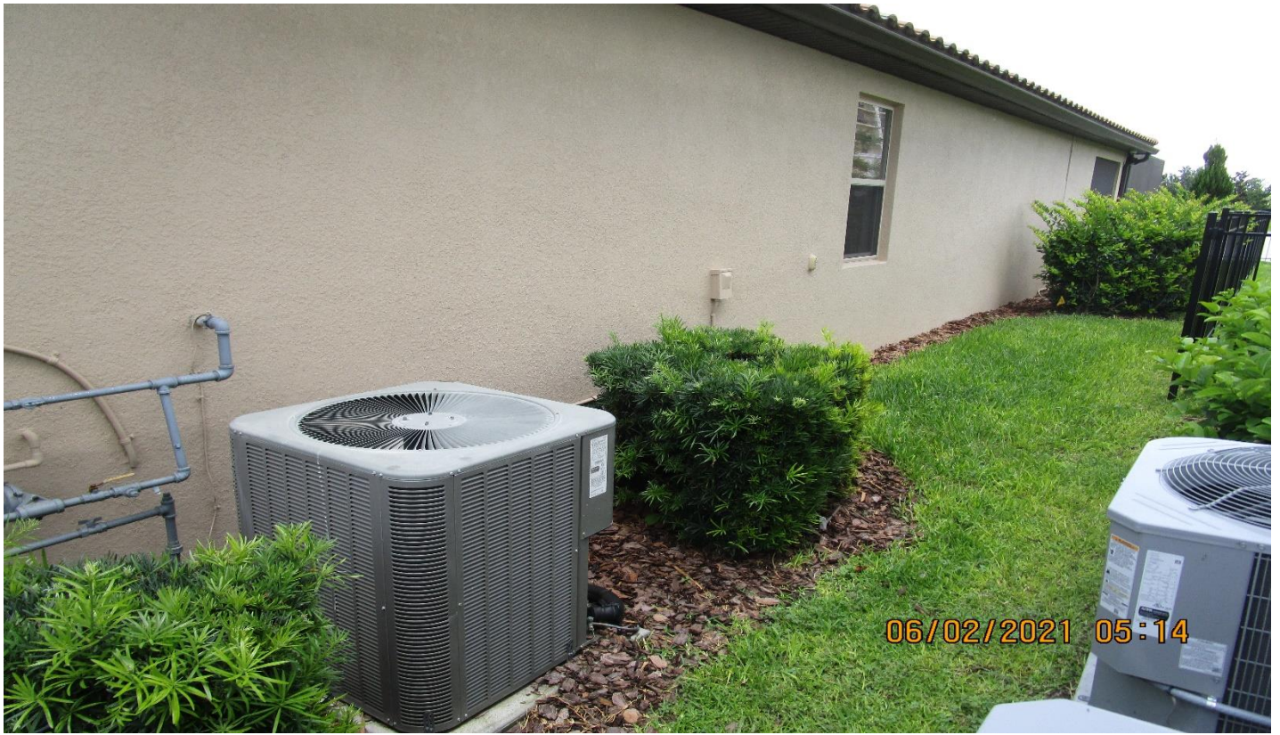
Side-Generator location facing north
