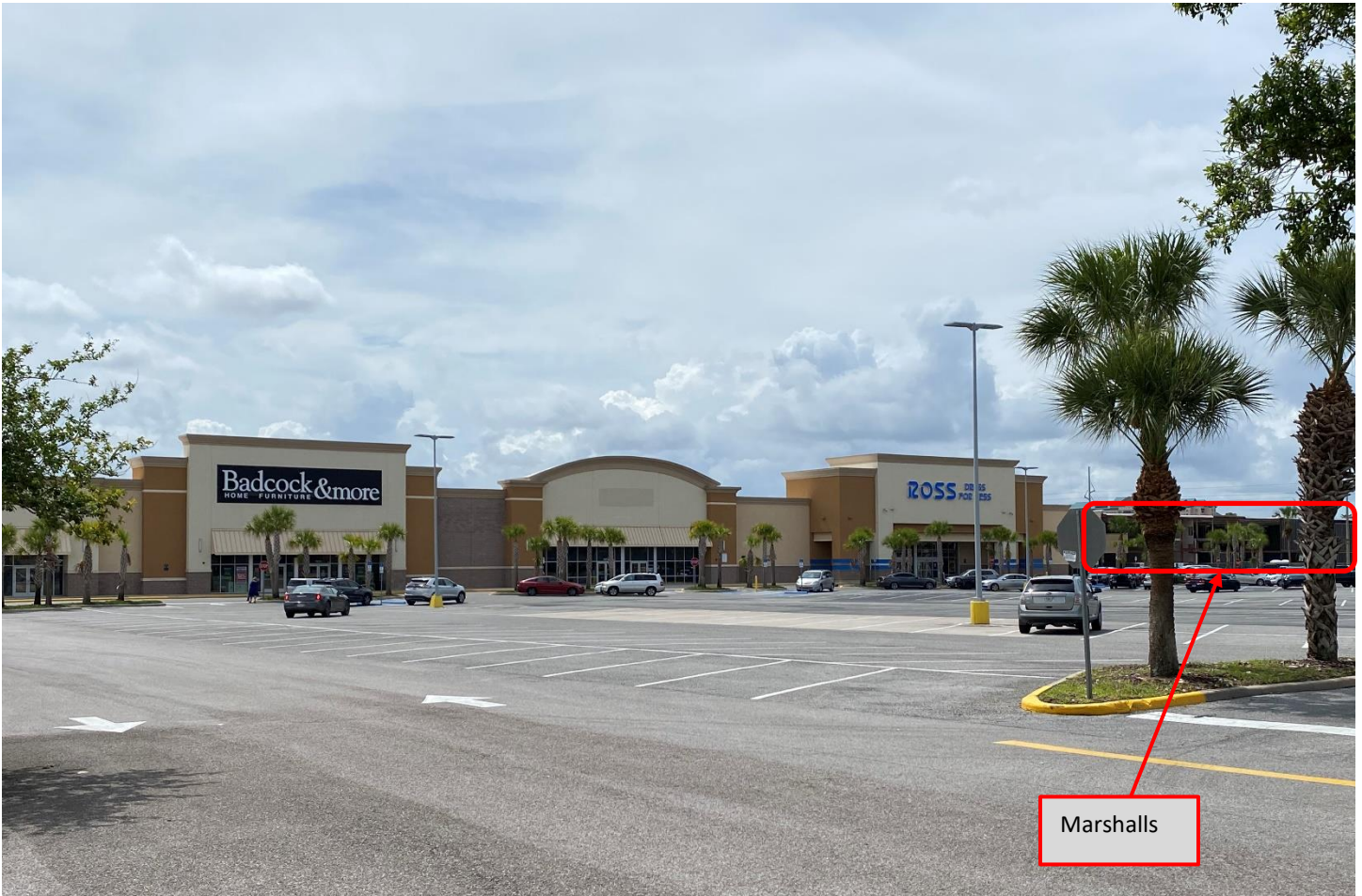
Front facing east (Taken approx. 115 ft. from center of S. Orange Blossom Tr.)
