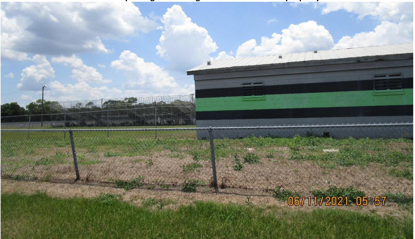
Drag strip stands facing west with Building 9 restrooms in foreground
