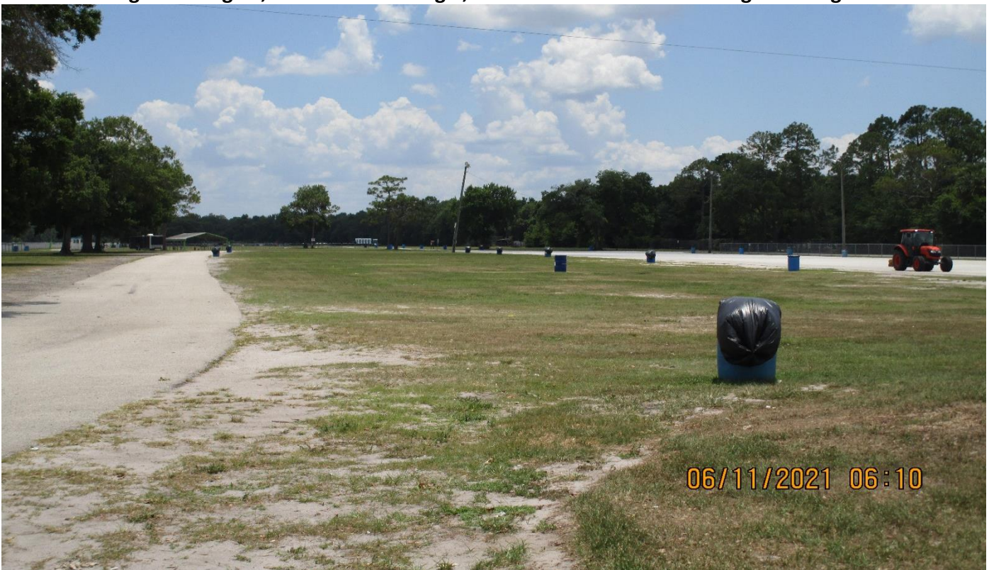
Overflow parking with new paved truck parking facing south with west landscape buffer to the right
